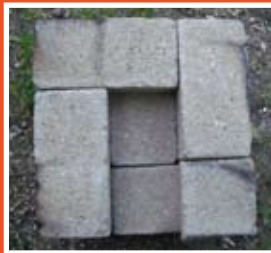
Brick Stove Layer 2
