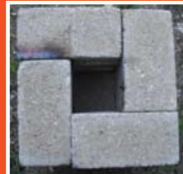
Brick Stove Layer 4
