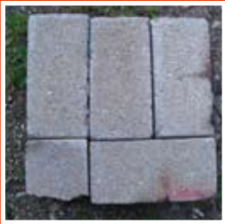
Brick Stove Layer 1
