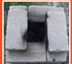
Brick Stove Layer 5
